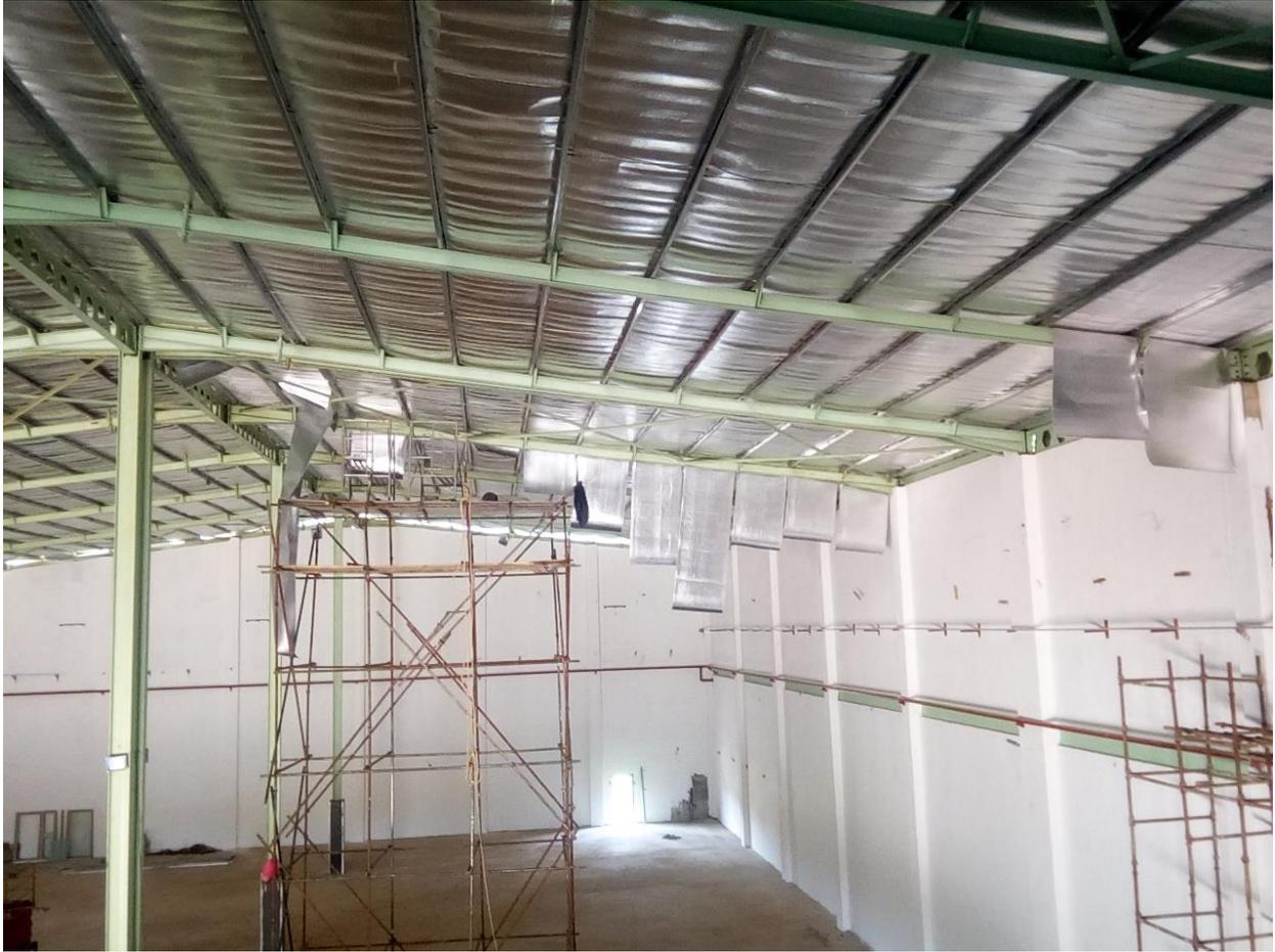
*Figure 3. Roof insulation- new layer being added*
