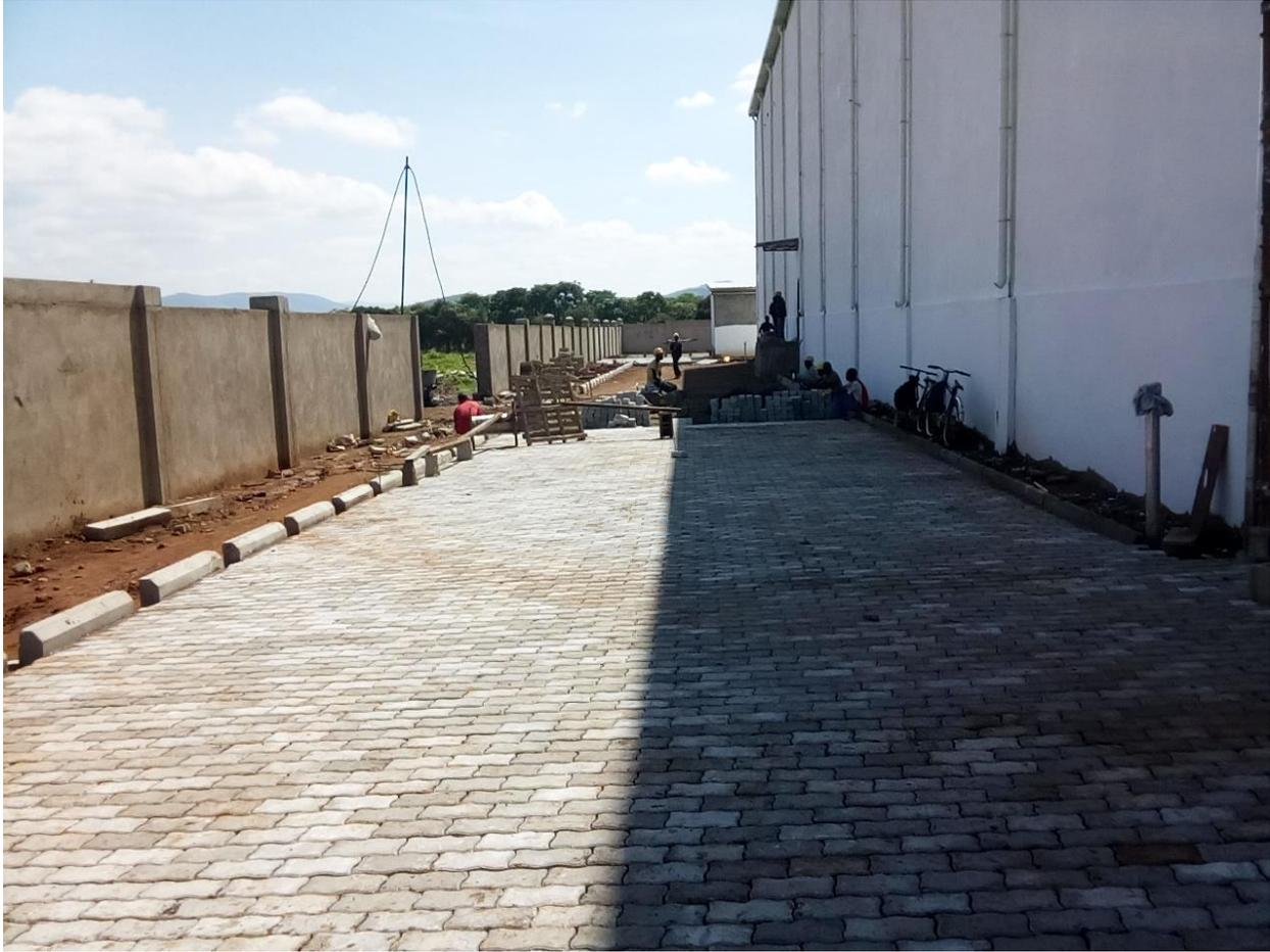
*Figure 4: Paving road works -Northern side of the warehouse building*
